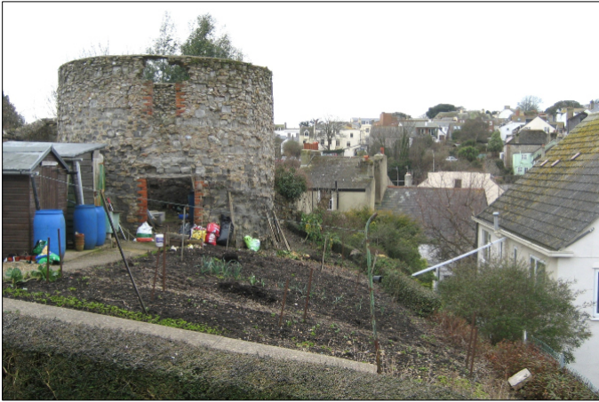
The Fleece Drying Stove above Coombe Street seen in 2010. A central stove heated wooden fleece drying racks under a conical slated roof.
