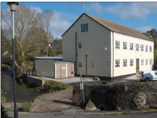
The New Factory. The river runs under the concrete bridge in the foreground
