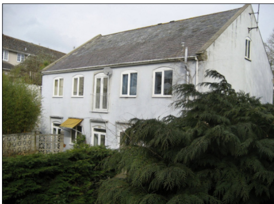
Old Silk Mill Flats, the surviving mill on the Old Factory site and the most recent part to be rebuilt. In this image it is converted, as Silk Mill Flats, viewed from across the river above Gosling Bridge (photo courtesy Martin Diplock).
